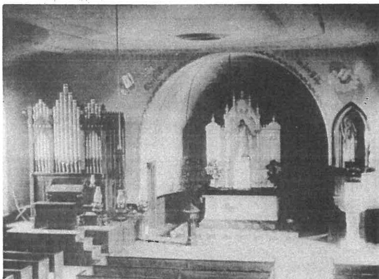
Inside of old church before renovation
